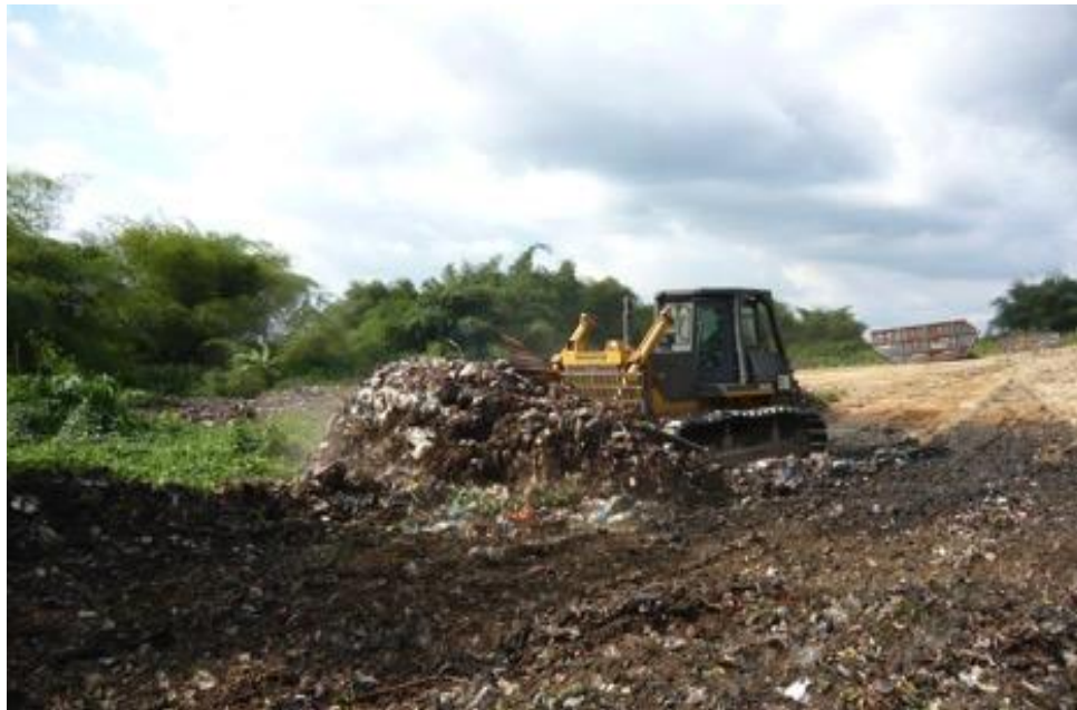
PUSHING AND SPREADING IN PROGRESS
