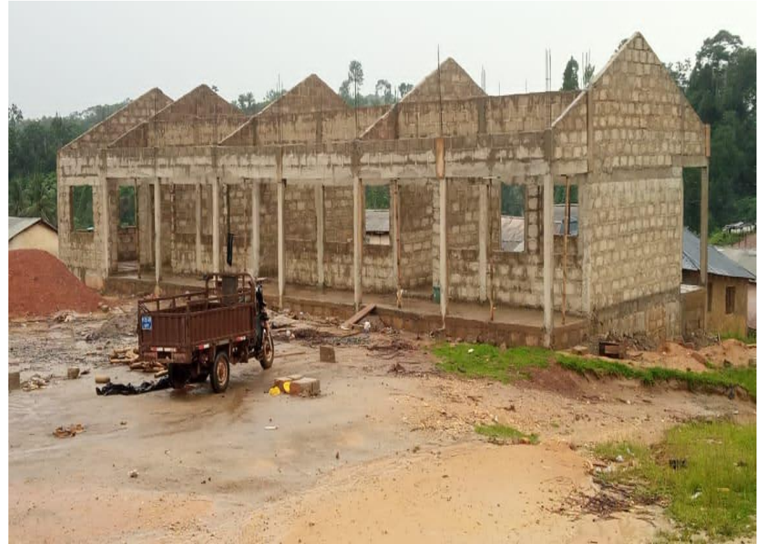
3-Unit Classroom Block at Obrayebona - Ongoing
