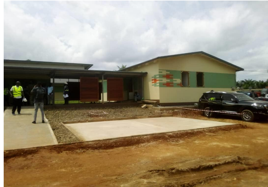
Remodelling and Expansion of the Mpohor Health Centre
