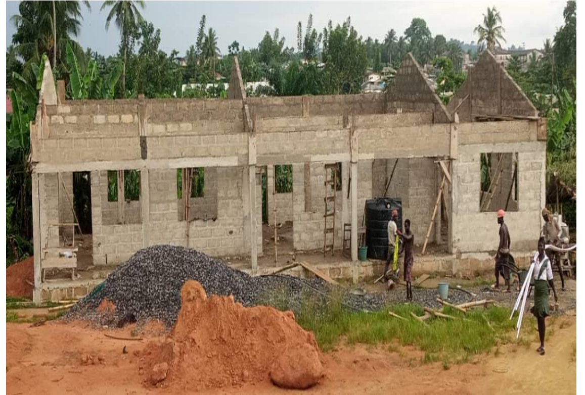
2-Unit Kindergarten Block at Mpohor SDA Basic School - Ongoing
